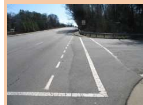
Highway 76: Intermittent paved shoulder
